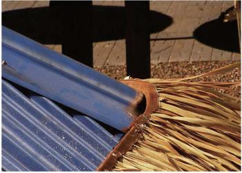
③ Cover the hips/corner with tiles bended to proper angle.
