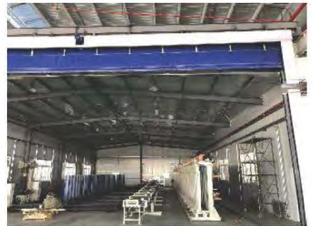
Tamp. Humidity control room
