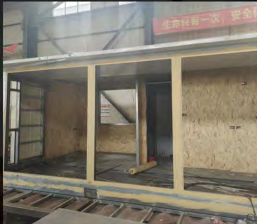
Reinforced structure with galvanized square pipes
