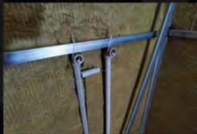
Manual insulation filling on all sides, up to 100mm thick
