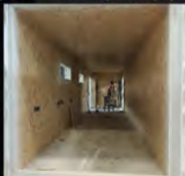
OSB for enhanced interior wall hanging capability
