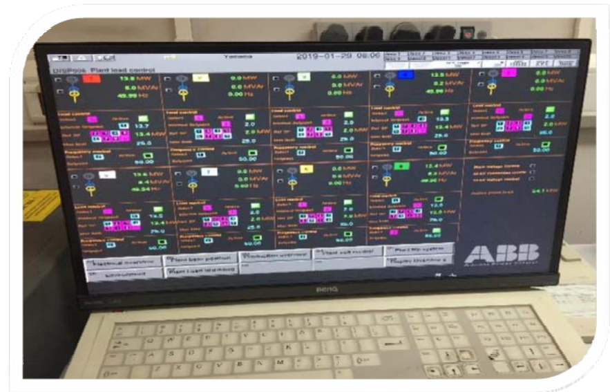
SIEMENS Gas Turbine Is Operated On ABB Advant Power Control
