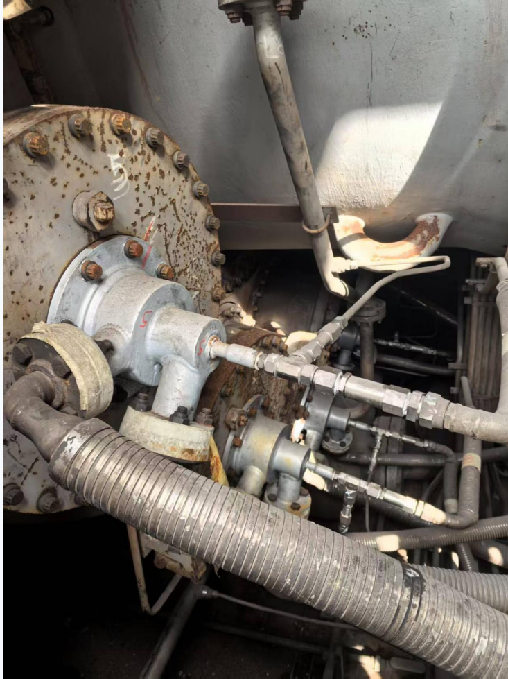
Combustion system (dual fuel)
